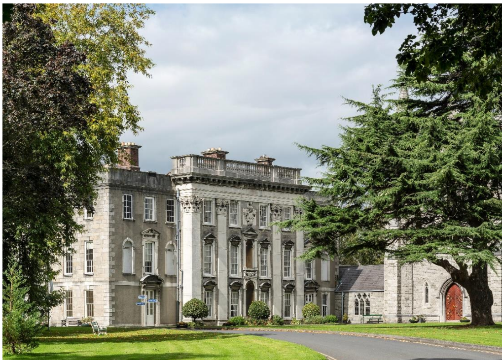
ALL HALLOWS' CAMPUS, DCU. HOME OF THE CHURCH OF IRELAND CENTRE
