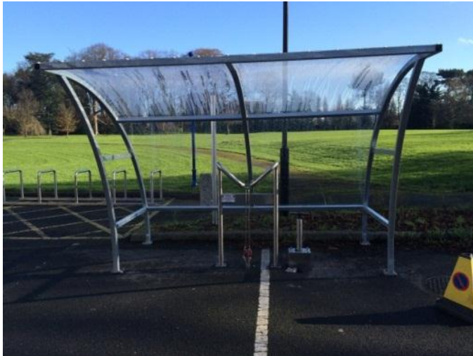
Figure 42: Cycle Maintenance Stands on All Hallows Campus
