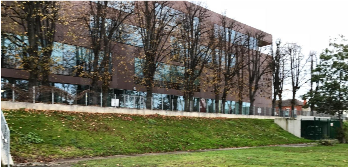
Figure 20: Sloped grass area from steps to boundary wall with Drumcondra road, also incl small area to left of steps.
