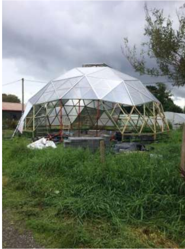
Figure 50: Grow Dome in DCU Community Garden under construction summer 2017.
